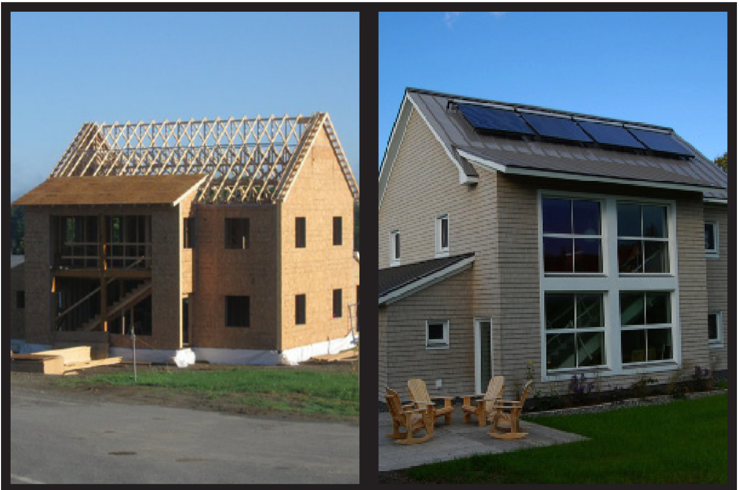
Photos: Before and after photos of Unity College's TerraHaus residence hall in Maine.
