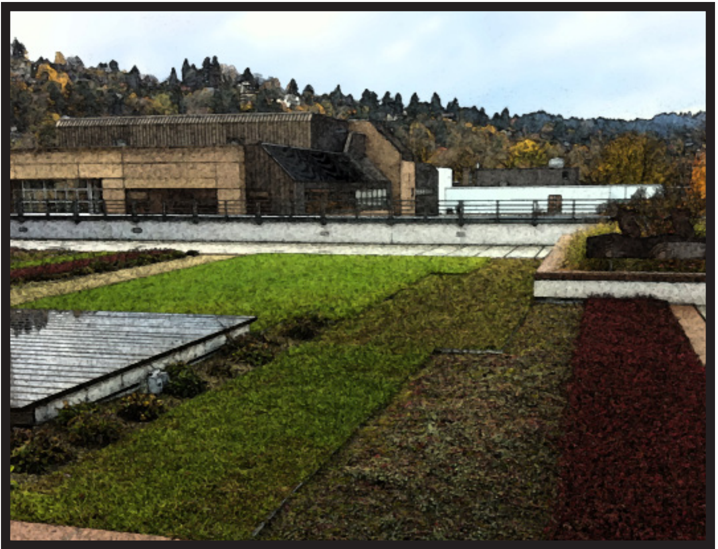
Photo: Green roof at Portland State University in Oregon.
